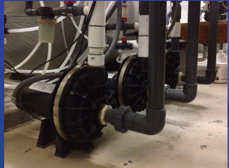
Chlorination Pump Replacement
